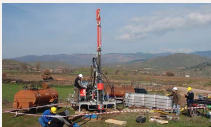
Drilling with the Ariana drill rig at Vein 9, Kiziltepe, Sindirgi Project.
